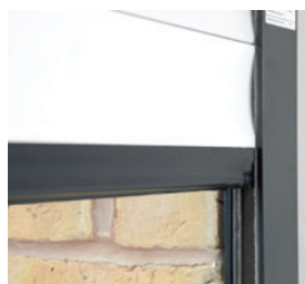
Heavy duty extruded aluminium guides secure the door at the sides.
